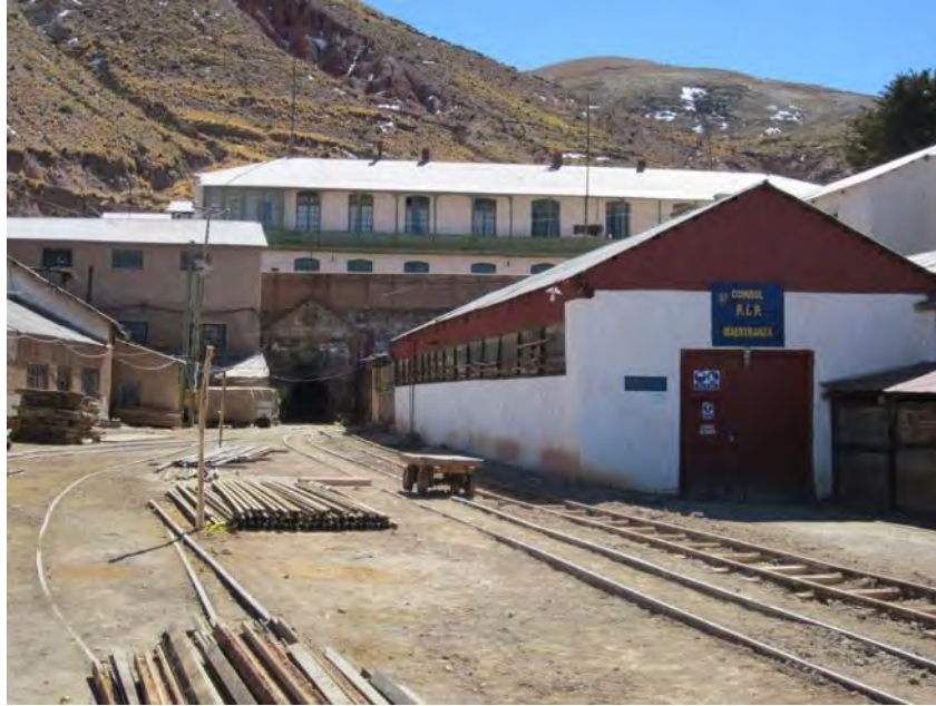
Figure 4.2: Pulacayo COMIBOL Operations Facility Used by Prophecy
