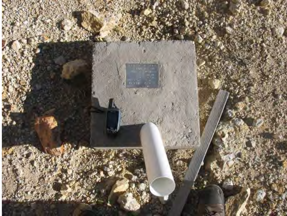
Figure 9.1: Typical Apogee Drill Collar After Completion of Hole
